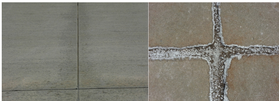
Figure 1. Joint “shadowing” (left) and eventual disintegration of concrete at joint (right).
