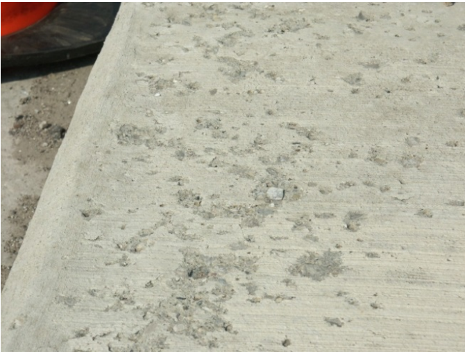
Figure 3. Concrete surface suffering deicer scaling.
